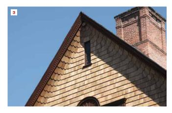
A photo from 1906 shows Naumkeag, in Stockbridge, Mass., with the original decorative shingling (1). Elaborate staging allows the crew to reach the gable peaks (2). The restoration crew replicated the curved scalloped shingles along the gable eaves (3).
